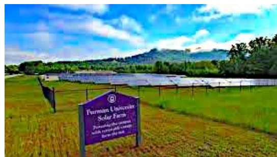
Furman University’s 7.4MW Solar Farm
